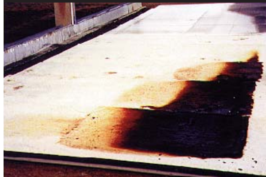
Sprinkler action: Internal inspection shows minimal contribution
