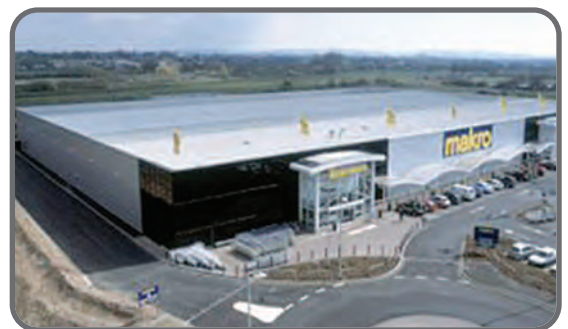
External: roof and walls
