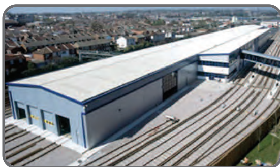
External roof panel application
